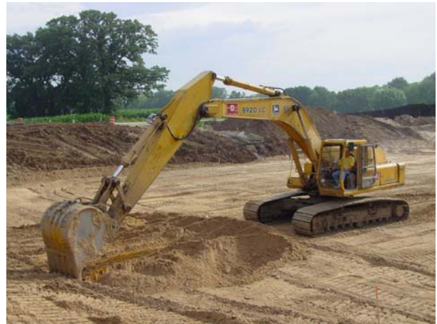
Preparing Native Soil Beneath Infiltration Basin
